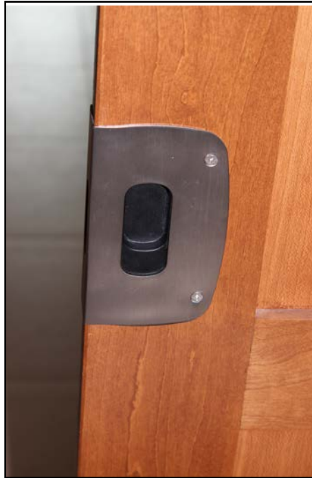
Figure 2-22: Pocket door hardware
