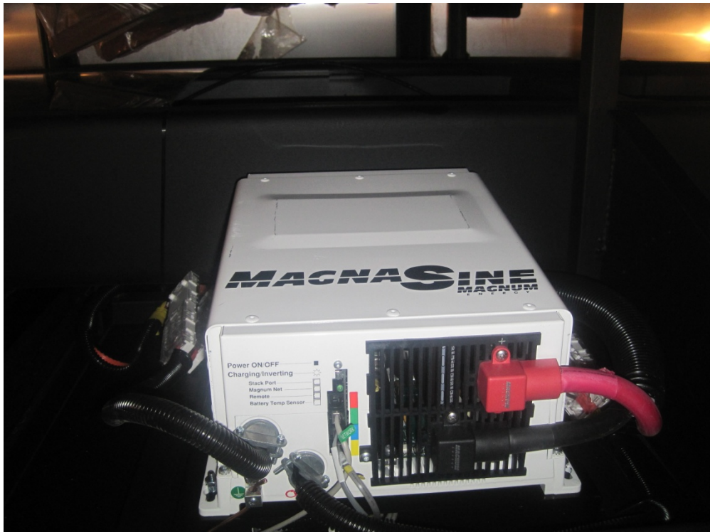
Figure 2-4: 2000 watt Sine wave inverter
