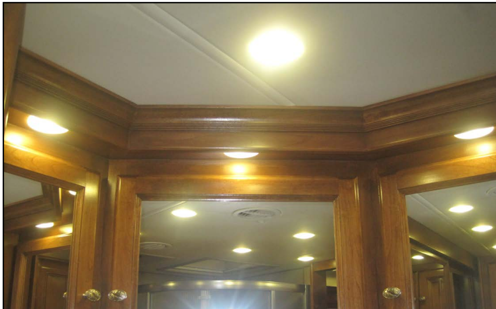
Figure 2-23: Crown molding in rear bath
